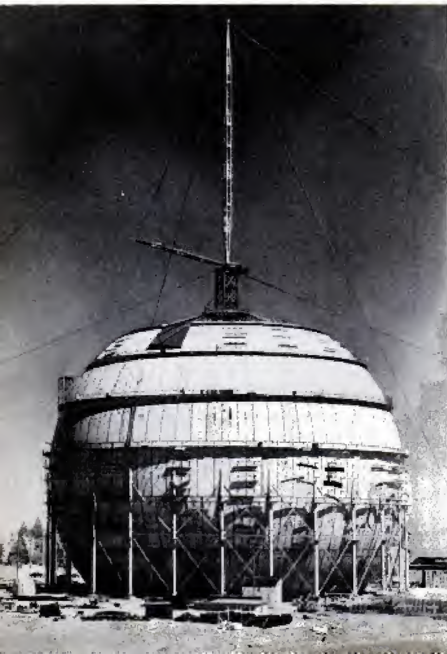
Five miles of welds on exterior of steel sphere were brushed with a soap solution to test for air leaks
